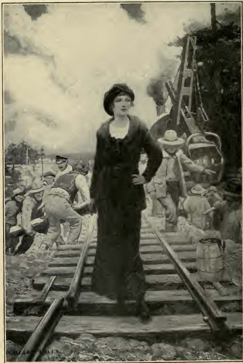
The single track railroad was indeed assuming form and a semblance of reality
